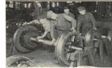
Coating with a fine suspension of chalk in alcohol
