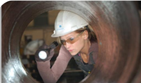
Visual inspection for surface cracks
