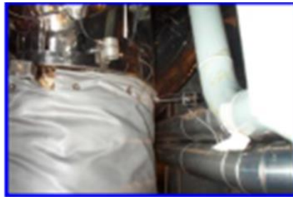
Pb Blanket in Nuclear Applications
