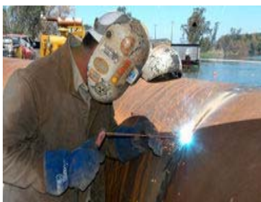
Examples of the MMA welding process
