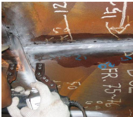
Magnetic particle inspection using a yoke.
