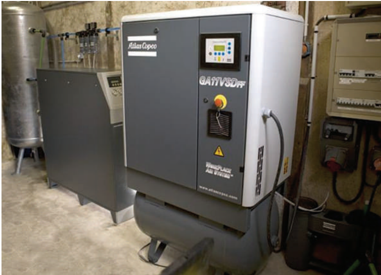
Example of a small rotary-screw compressor. (Photo courtesy of Atlas Copco.)
