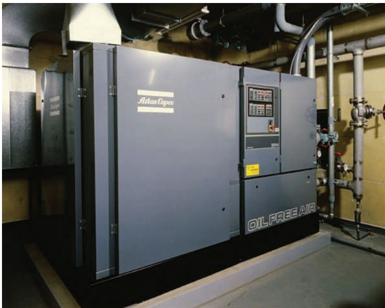
An example of a big rotary-screw compressor (old-fashioned oil-free type). (Photo courtesy of Atlas Copco.)
