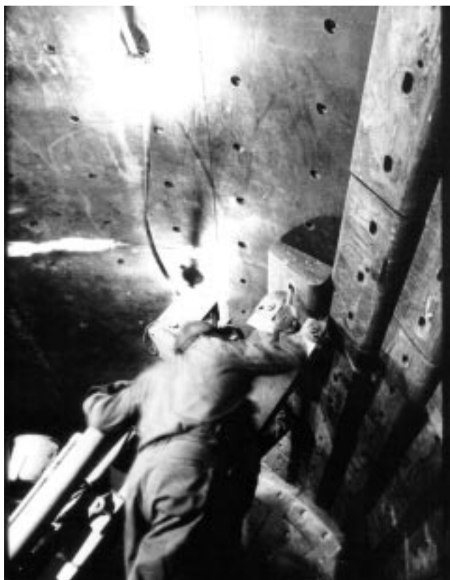
Fig. 10.18. Installation of Ni-Hard 1 (ASTM IA) liner plates in a ball mill. (Courtesy of NiDI)
