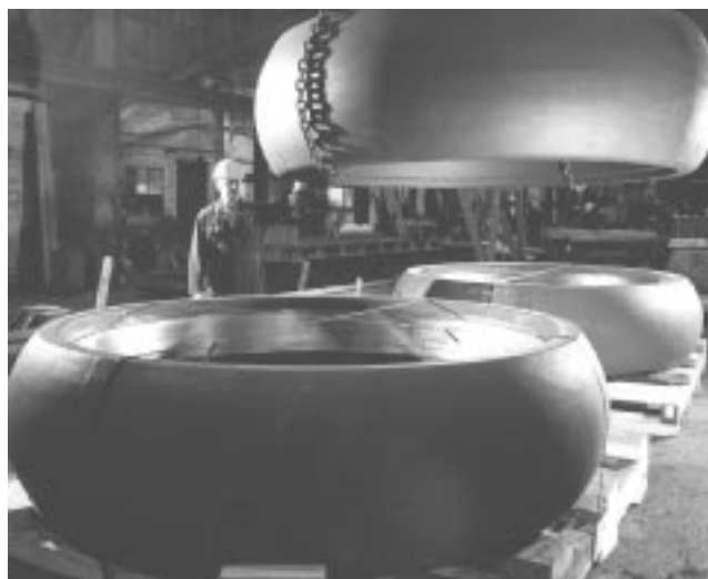
Fig 10.24. High-Cr (ASTM IID) coal-crushing replacement rollers. The inside bearing races have been machined and are ready for field installation. (Courtesy of Firth Rixson Castings)
