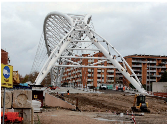
Figure 2. The Garbatella bridge seen from its western side. AE monitoring was carried out at the base of the single eastern "leg" here shown in the background.
