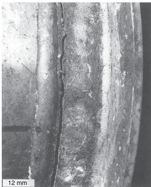
Figure 11.8 Photograph showing a severe stress corrosion crack running along the HAZ in a cast CF8M (type 316) flange welded to a pipe formed from sheet 316. Cracking was due to weld sensitization and subsequent corrosive attack. Source: Chakrapan (1992). Used with permission of ASM International.
