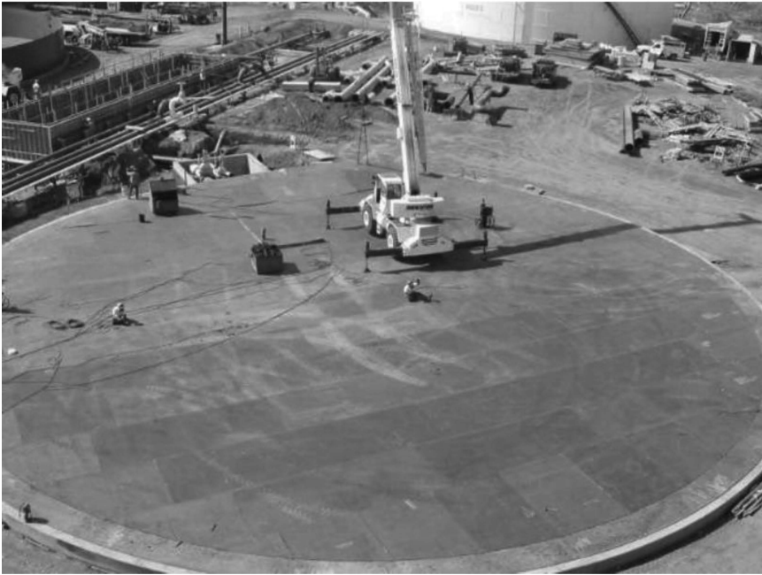
Tank bottom in progress.
