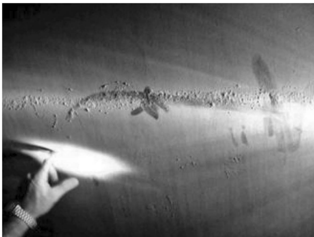
Blistering where a stiffener was welded on the other side of the plate.
