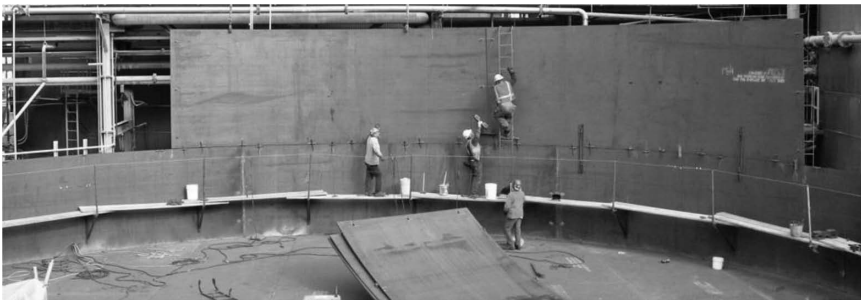
Erection of second shell course in progress.
