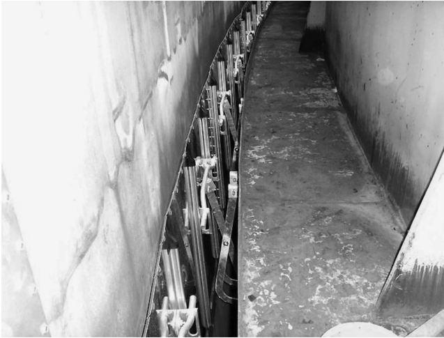
Installed shoe arm and counterweight arm.
