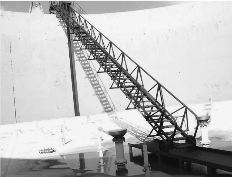
Rolling ladder and antirotation device.
