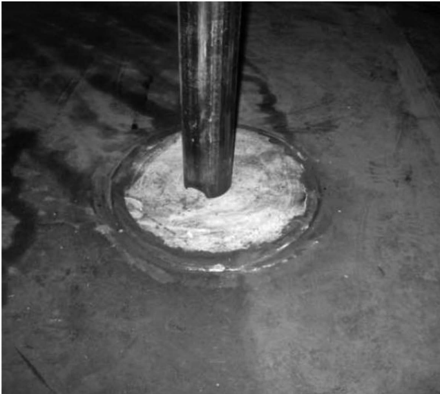
Reinforcing pad for roof leg.
