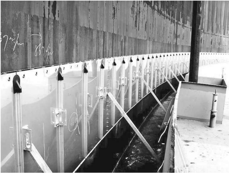
Shoe plates after installation.
