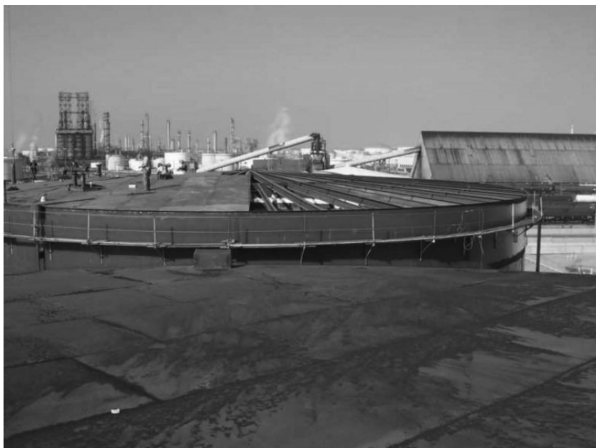
Supported roof partially completed.
