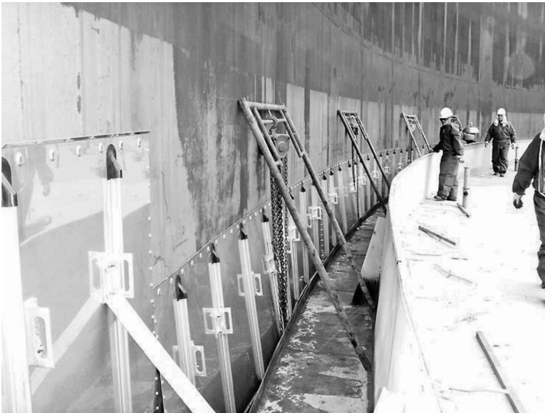
Shoe plate attachment works.
