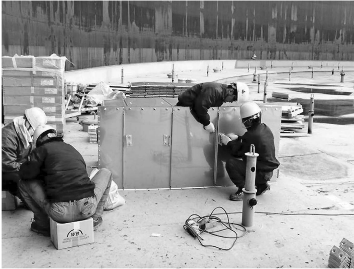
Preparation works for attaching shoe plate.
