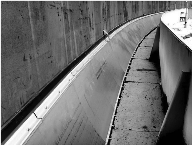
Secondary seal system.
