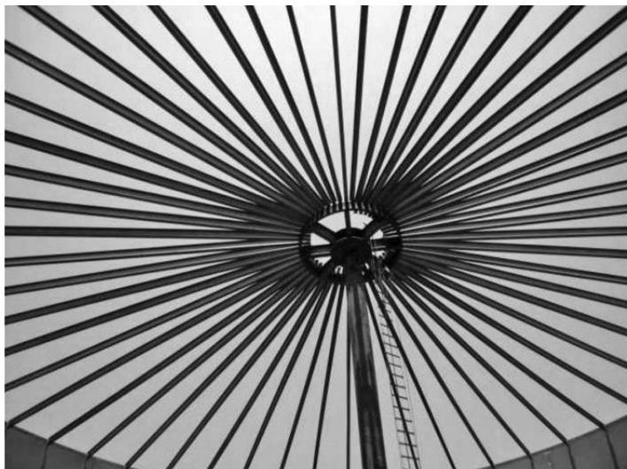
Roof rafter construction in progress.
