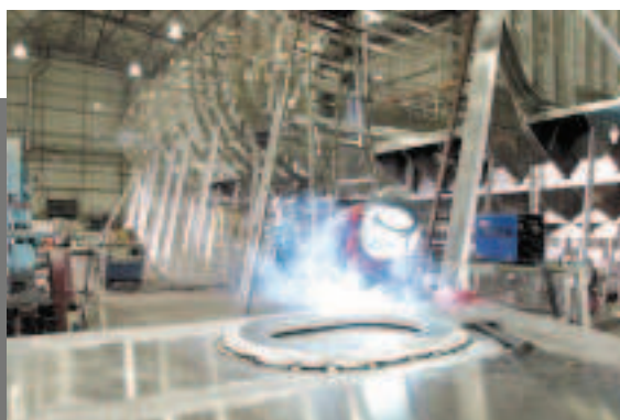
WELDING A HATCHWAY FRAME
