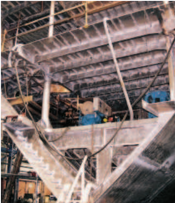
LIFTING ALUMINIUM SUB-ASSEMBLIES
