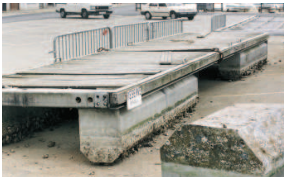
MARINA PONTOON AND FLOATS MADE OF 5754
