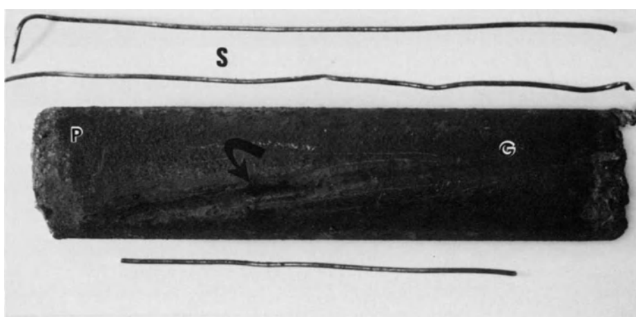
Fig. 17-2. Galvanic or bi-metallic corrosion between the stainless-steel capillary tubing (S) and the carbon-steel pipe (P) caused the formation of the spiral groove (G) and, ultimately perforation (arrows) and loss of pressure.
