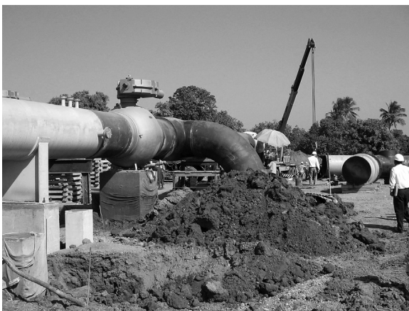
FIGURE 2-8-3 Typical construction site — Note the main line valves welded to the pipeline.
