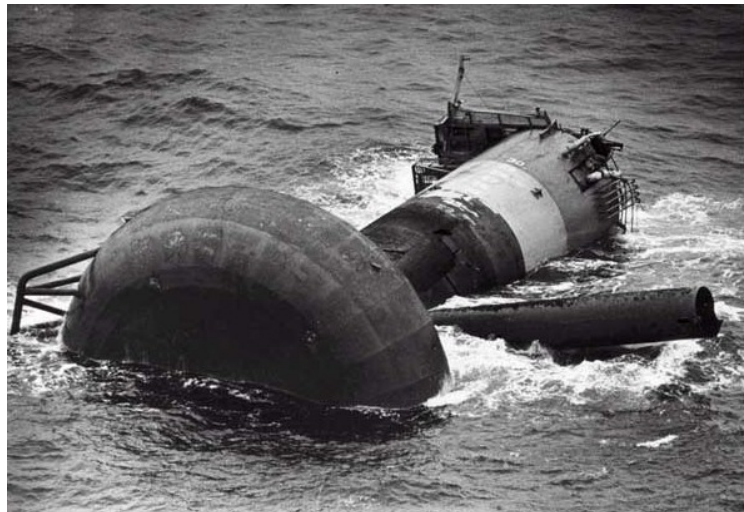
Fractures on the bracing of the Alexander L. Kielland rig
