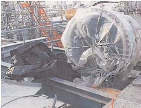
Pipe opening where a confined space was inadvertently created
