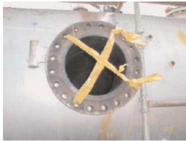
Picture of the separator after the incident, with inadequate physical barrier and lack of signage.
