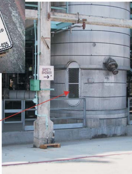
Vessel skirt manhole is closed by a locked door
