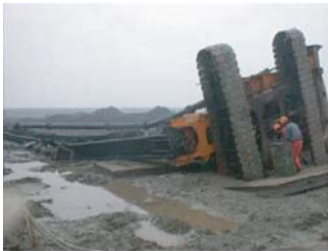
Fallen pile-driving rig
