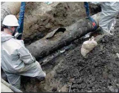
Removal of ruptured pipe section
