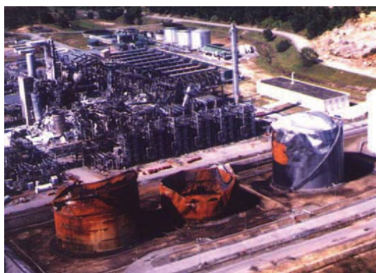
Figure 49 Explosion on a cryogenic distillation column.
