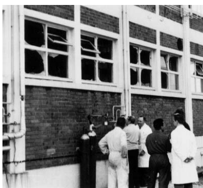
Figure 50a Damage caused by flexible hose rupture.
