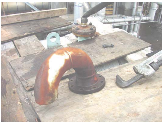
Figure 57a Vent and water hose installed.
