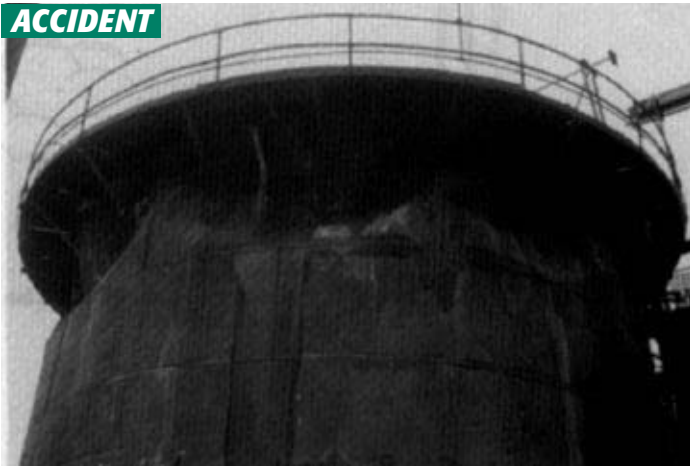
Figure 10 A vacuum vent and one open hatchway were not enough to prevent damage when steam condensed and pulled in the top two courses of this 35 ft (10 m) diameter by 21 ft (6 m) high wash tank.
