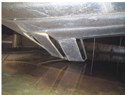
Figure 42b Collapse of a tank with internal floating roof due to excess weight applied.
