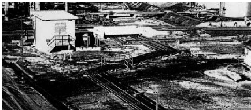
Figure 16b Projection of bitumen over pipe-racks.
