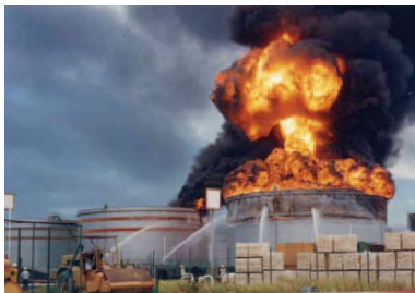
c. Adjacent tank beginning to burn.
