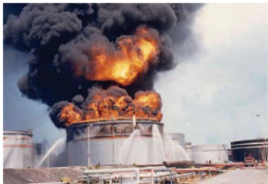
b. Tank ignited by foam application.
