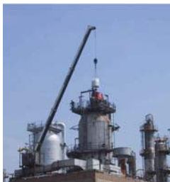
Reloading of a reactor using 'big bags'
