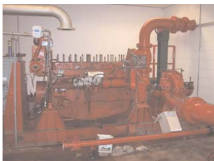
Overhaul of a diesel fire pump.
