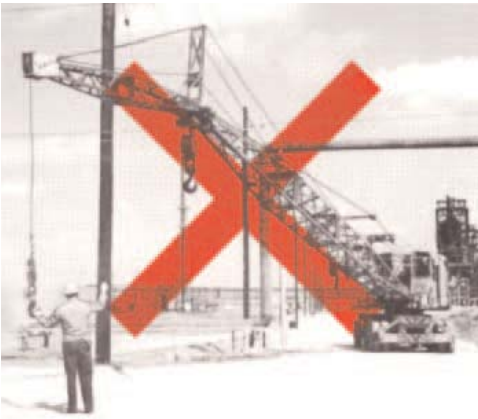
Figure 68 When a crane boom is moving near overhead electrical lines, don't grab the hook or touch the crane! Wait until you are sure the boom has stopped a safe distance from the wires.
