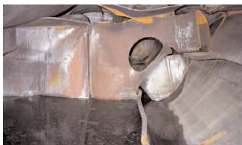
Cargo tank sump with feed pipe (left), submerged pump and bilge pump. The green arrow shows the supposed site of the explosion (between the wall and discharge pipe).
