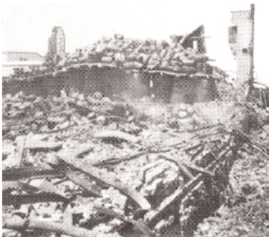
Figure 45 Proper grounding would have prevented this fire.
