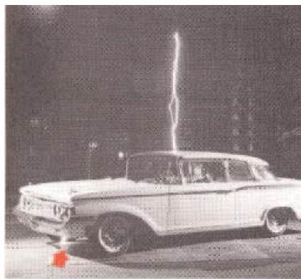
Figure 25 Demonstration showing that lightning (in this case, a 3 million-volt stroke from high-voltage generator) will not harm a person inside an automobile. Note the current flowing to ground near the right front tyre.
