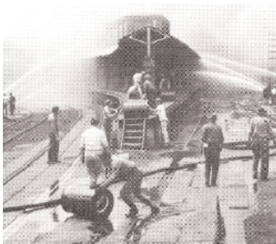
Figure 44 Barrel-house fire caused by poor electrical grounding.
