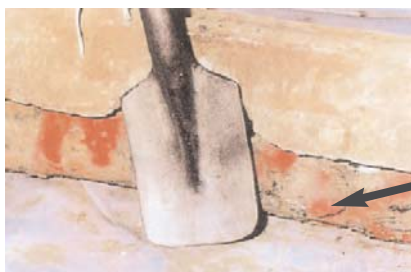
Small pneumatic clay spade fitted to the damage site.
