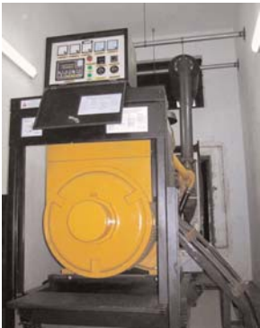
Diesel generator in two hours fire rated room with fuel tank in adjacent room.
