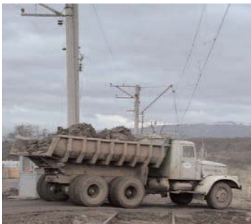
Railway crossing. Metal pole contacted the overhead power line located on the right hand side of the photo. The truck crossing the railway line provides scale. The overhead power line is approximately 5.7 m above the ground. The metal pole measured 6.0 m in length.
