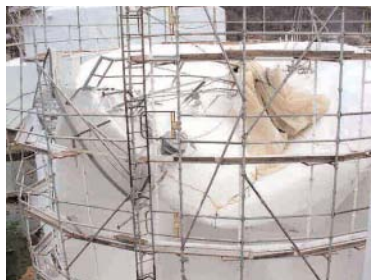
Pressure/vacuum safety valve of the tank was covered with a plastic bag during painting, causing the tank to be sucked in during a product transfer.
