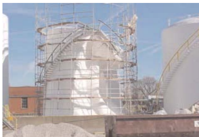
Pressure/vacuum safety valve of the tank was covered with a plastic bag during painting, causing the tank to be sucked in during a product transfer.
