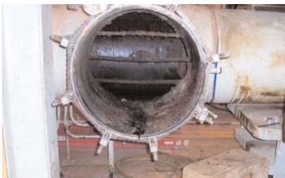
View of the 28 inch (71 cm) pipe
