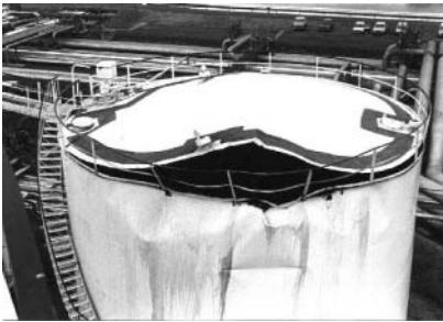
Another incident where a storage tank fails at shell-to-roof seam (fish mouth) due to overpressure.
