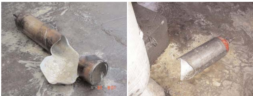
The two compressed gas aluminium cylinders that ruptured due to flame impingement.
