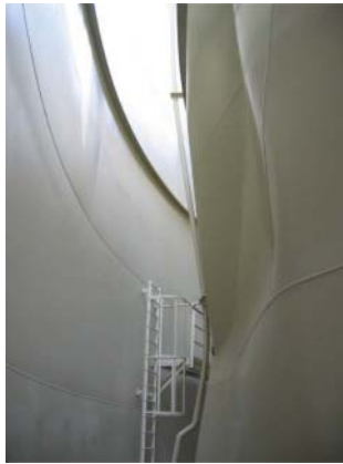
Another incident where a storage tank fails at shell-to-roof seam (fish mouth) due to overpressure.
