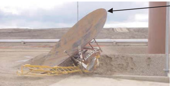
The tank roof and its associated structure on the ground.
