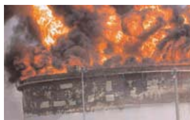
Fire once the roof lost buoyancy
