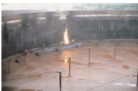
Rimseal fire at an early stage
