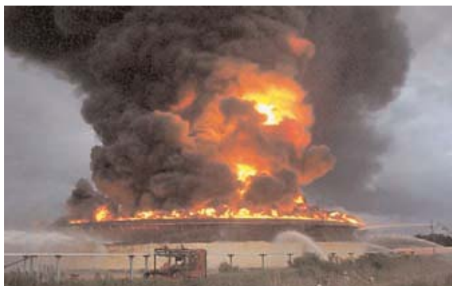
This full surface 83 m (270 ft) diameter tank fire was successfully extinguished using mobile equipment (application rate roughly 8.8 l/m 2 /min (0.21 gpm/ft 2 ), no wind or rain)
