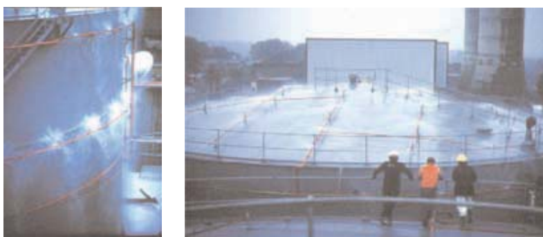
Tank shell and roof waterspray tests
