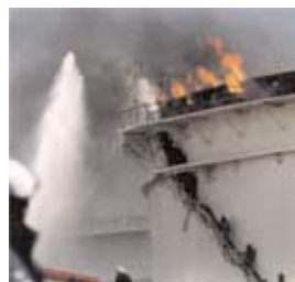
Attack of a rimseal fire from stairway—see how much manpower is needed to deploy flexible hoses when there is no fixed dry risers.
