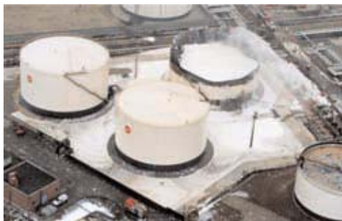
Example of partial fold-in of a tank shell. The liquid level is well visible as the product kept the paint cool and intact.
