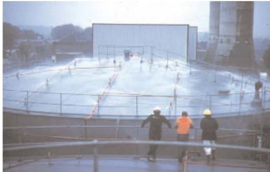
Tank shell and roof waterspray tests
