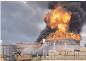
c. Adjacent tank beginning to burn
