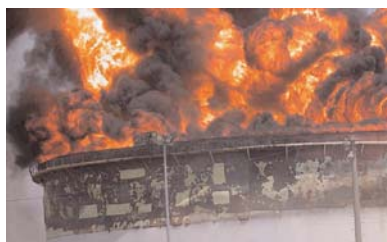
Fire once the roof lost buoyancy
