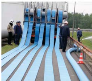
8 lines of 8" hoses layer truck
