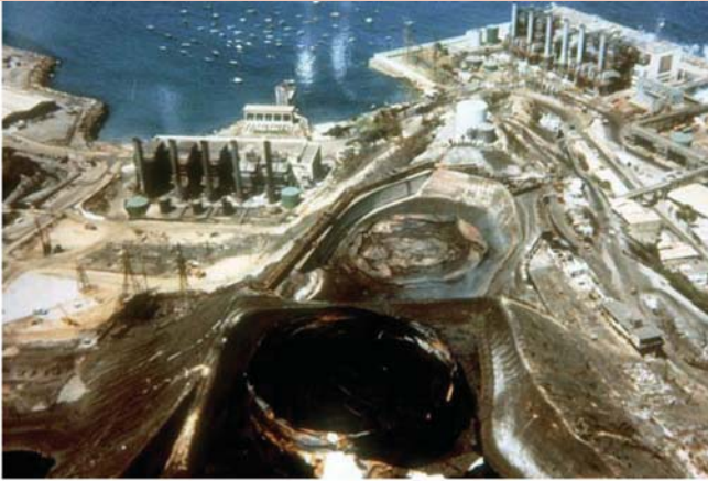
Tank 8 is in the foreground, tank 9 is in the middle of the picture. Note the steep hill where the tanks are located and unique access road below.
