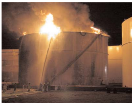
Fires at the vents are very difficult to tackle. This 95 ft (29 m) gasoline tank fire was extinguished by using foam and three of the vents were 'shot out' utilizing dry chemical (Hydro-Chem™ type).
