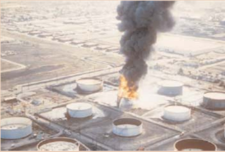
Good spacing prevented escalation of this tank fire to adjacent equipment.
