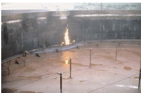
Rimseal fire at an early stage
