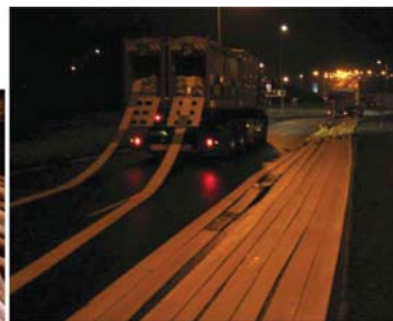
Laying of 6" hoses from containers
