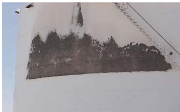
Signs of an internal rimseal fire that ignited after this tank was exposed to radiant heat from another tank fire.
