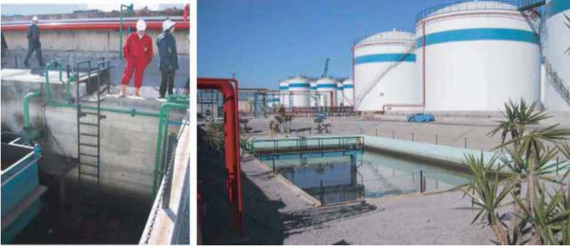
Open water treatment pits present the hazards of gassing and drowning. Note: No life jackets available.
