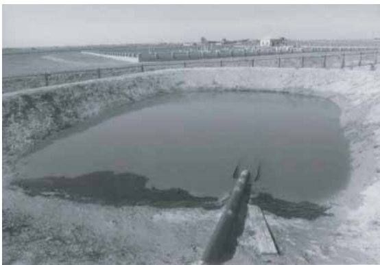
Earth pit used to collect oily water for recovery—possible seepage into the ground
