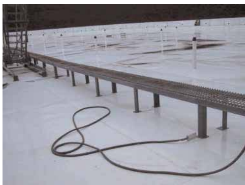
Bonding of floating roof
