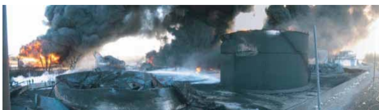
View of terminal damage 24 hours after the explosion
