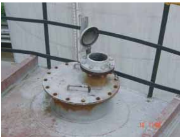
Sampling hatch is left open—poor practice
