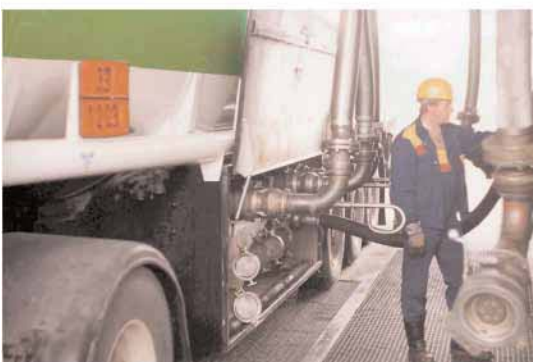
Bottom loading of a road truck. End of hose fitted with a dry break coupling
