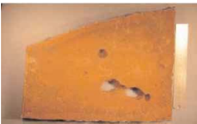
Holes in floor plate found local to tank inlet nozzle
