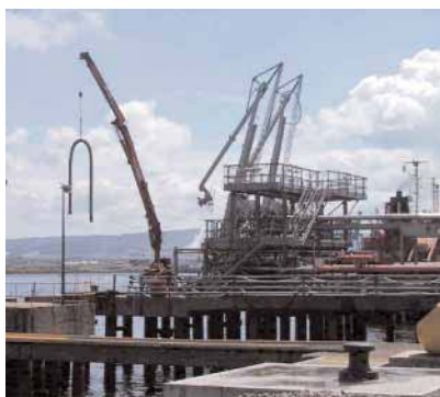
Use of steel wires in direct contact with hose should not be permitted. Bent to a radius less than that recommended by the manufacturer.
