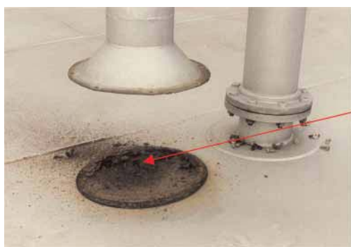
Rust partially blocks a screen mesh on a fixed roof tank's open vent
