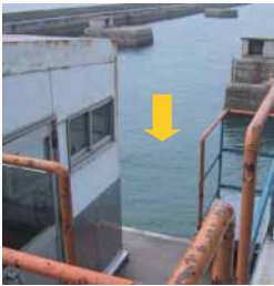
Missing handrail
