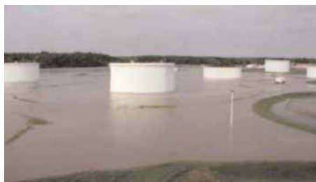
Flooded tank farm
