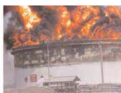
Fire once the roof lost buoyancy
