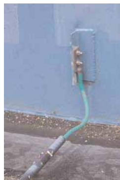
Tank grounding/earthing
