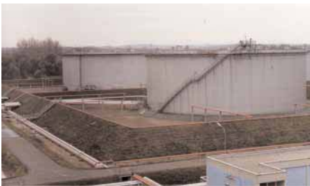
Typical floating roof tank farm with each large tank having its own individual bund/dike.
