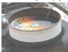
Roof covered by product.
