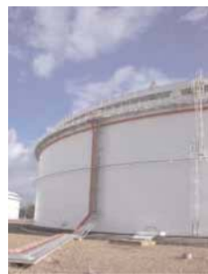
Example of a crude floating roof tank contained in metallic bund.
