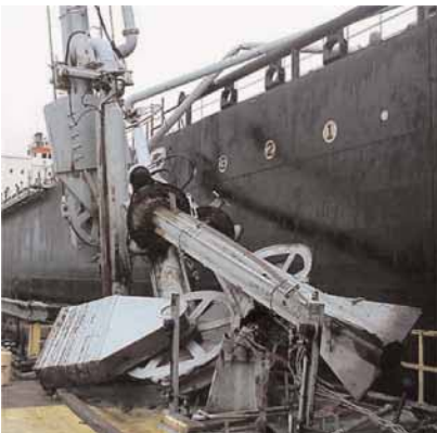
Result of loading arm going outside its safe operating envelope.
