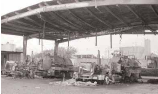
Burned out vacuum trucks
