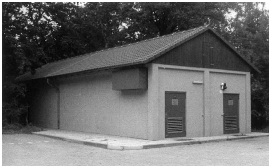
Figure 8.7 Multifunctional cubicle (MUK).
