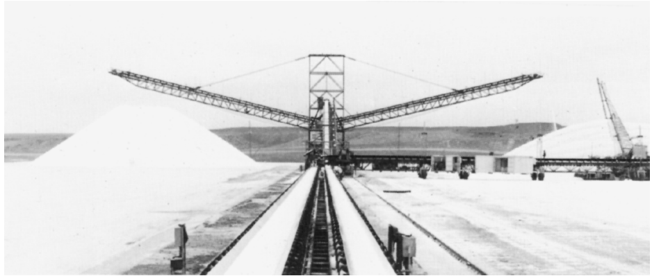
Figure 1.11 Double-winged stacker discharging into high-capacity stockpiles on either side of the feeding conveyor.
