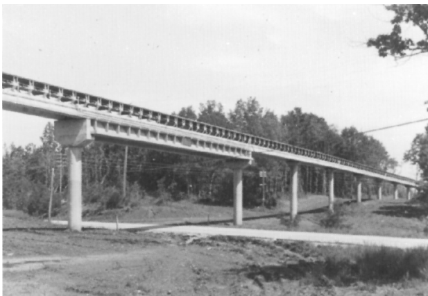
Figure 1.22 Overland conveyor system utilizing a concrete support structure provides a pleasing appearance blending with the landscape.
