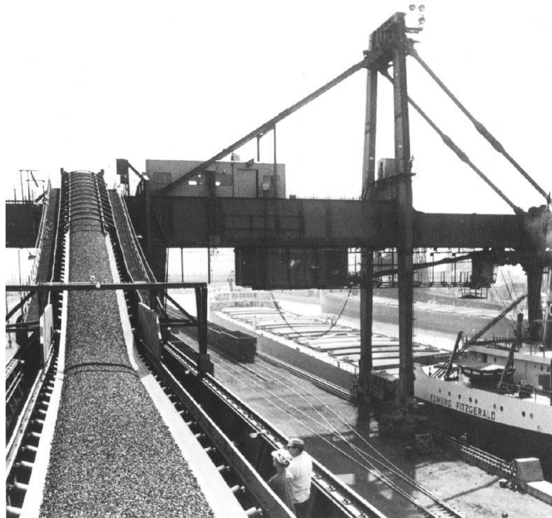
Figure 1.2 96-inch conveyor at high-capacity coal-loading facility.
