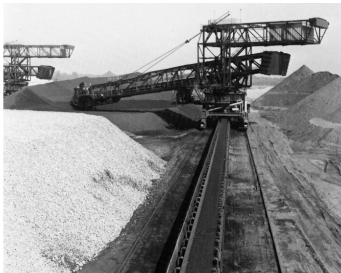
Figure 2.22 Bucket wheel reclaimer with wheel at end of boom.
