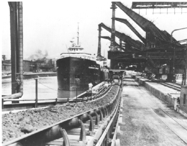
Figure 1.15 Rail-mounted ship unloaders feed 60-inch conveyor system at steel company.
