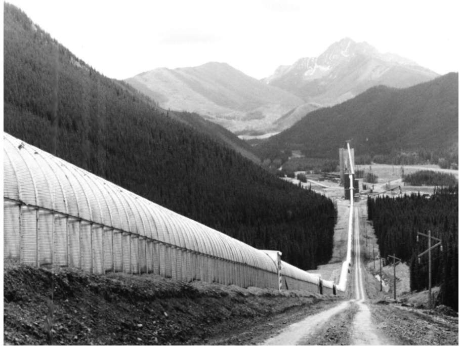
Figure 1.3 Regenerative conveyor lowers coal across existing terrain in direct path from mine.
