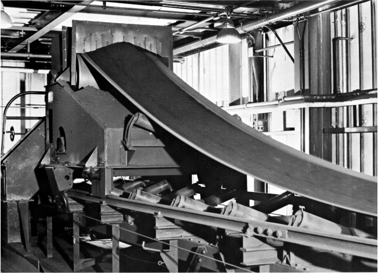
Figure 12.29 Typical motor-driven belt conveyor tripper.
