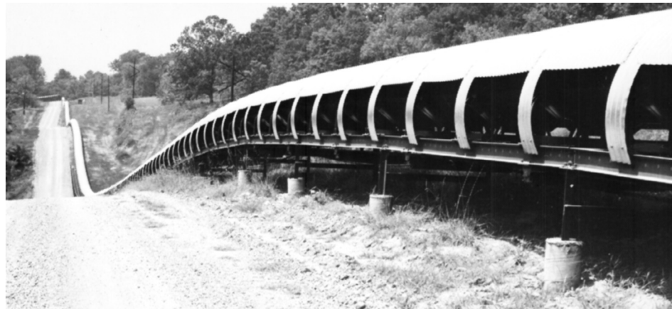
Figure 2.19 This overland conveyor following the natural terrain has an undulating profile with several concave and convex curves.
