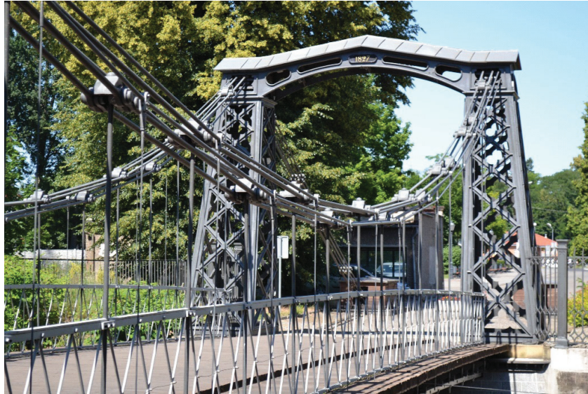
Fig. (2). The bridge, cast from cast iron elements in Ozimek, Poland, 1827 year; Courtesy Marcin Widera, (Local Administration of a Commune Council in Ozimek).
