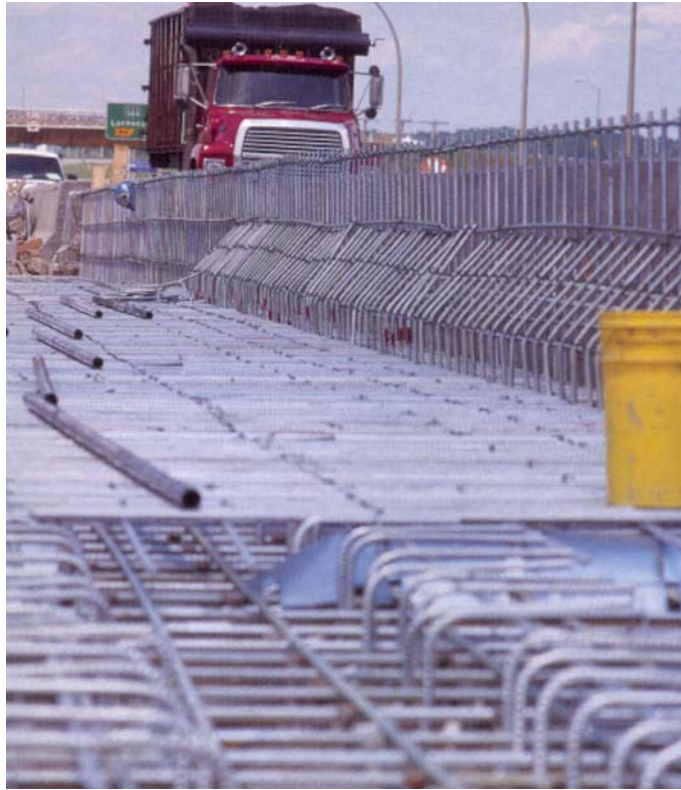
Figure 9.1 50 million tonnes of carbon steel is used annually to reinforce concrete. Stainless steel, either austenitic or duplex, is no more expensive, over a 100-year life of a bridge. (From Nickel, Vol. 14, No. 1, p. 15, 1999. Reprinted by permission, The Nickel Development Institute.)
