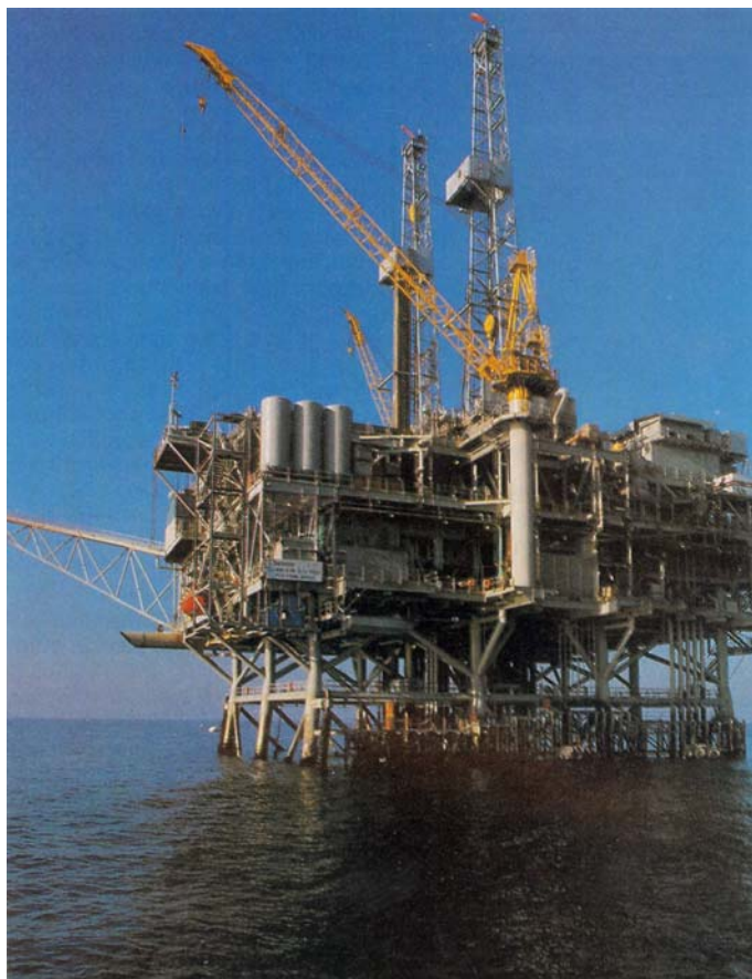
Figure 10.7 California offshore drilling platform coated with inorganic zinc and vinyl topcoats after 15 years of service. ( From C.G. Munger, MP, Materials Performance, Vol. 32, No. 9, p. 41, 1993. Reprinted by permission, NACE International. )
