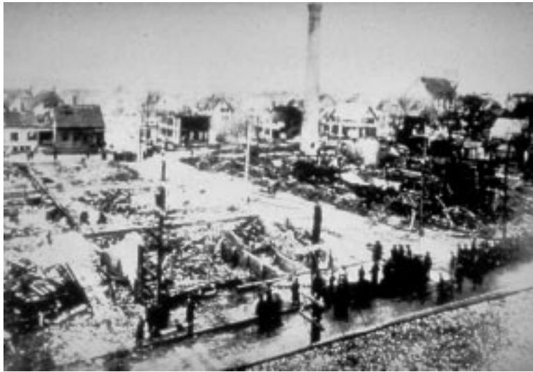
Figure 1.2b R.B. Grover Shoe Company. March 20, 1905, after explosion.
