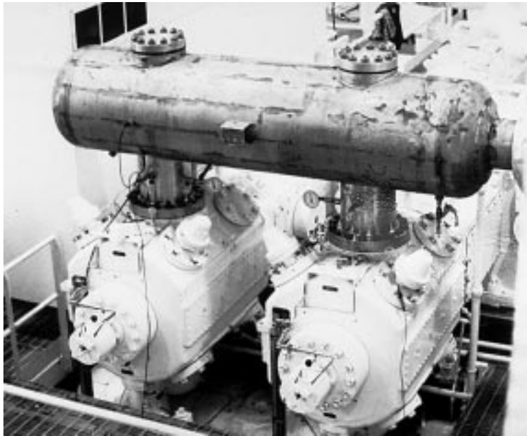
Figure 2.2 Reciprocating compressors are sources of vibrating pipe.
