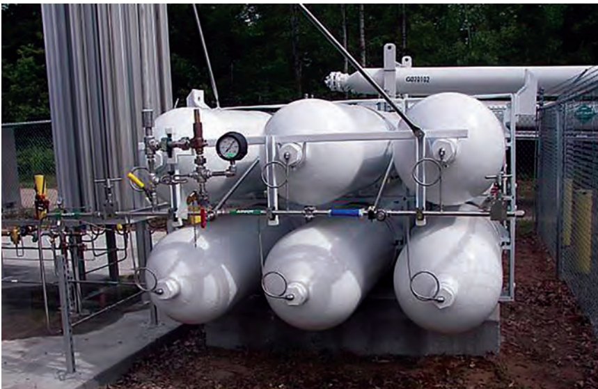
Fig. 4.15 Typical arrangement of six-pack of high-pressure gas storage hydril tubes. Courtesy of Air Products and Chemicals, Inc.
