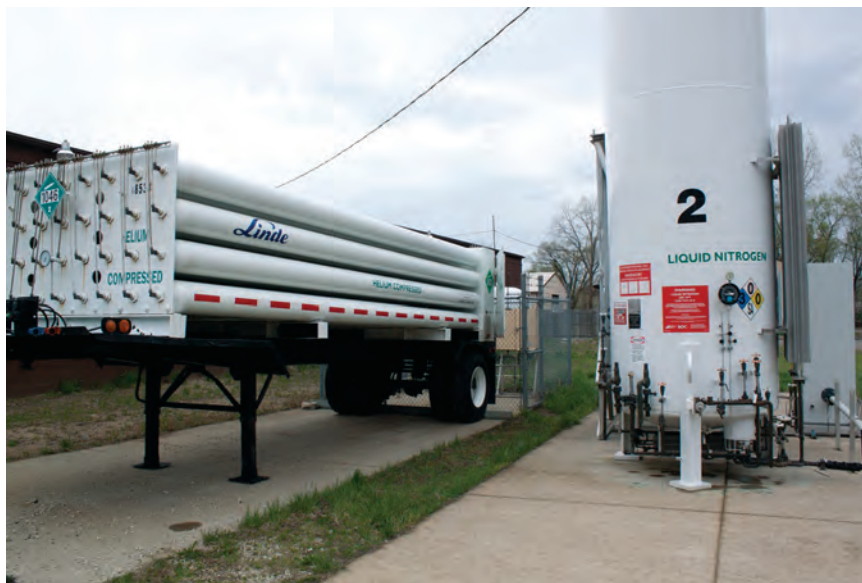
Fig. 4.11 Gas supply systems for cold spray processing. Helium from the tube trailer on the left; nitrogen from the liquid nitrogen pump system on the right. Courtesy of ASB Industries, Inc.
