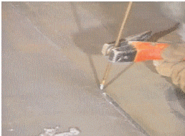
Figure 3.22(a): Manual air carbon arc torch.
