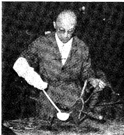
b. Pouring. Note the tilting of the mold at the beginning of the operation.
