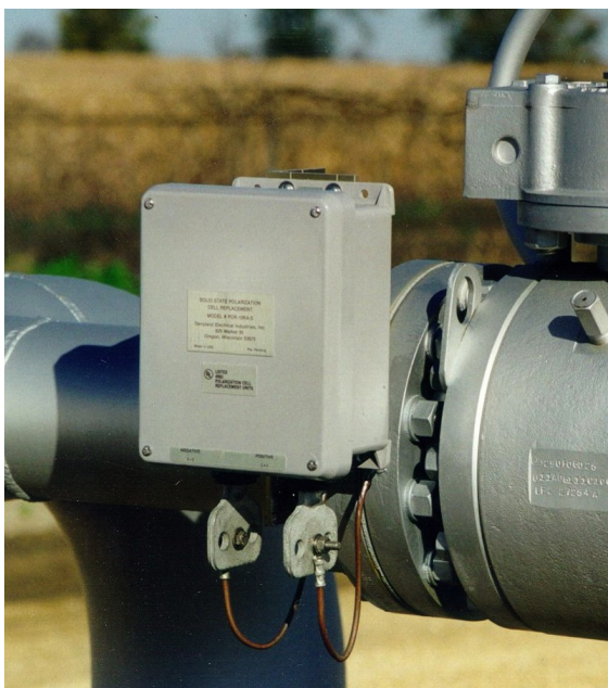
Figure 3-75: Solid State DC Decoupling Device
