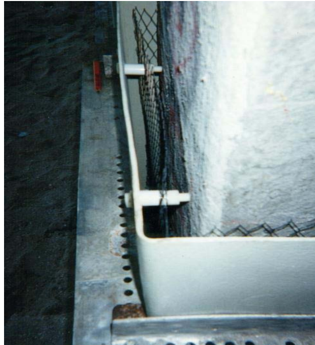
Figure 9.3 Titanium anode in a pile jacket
