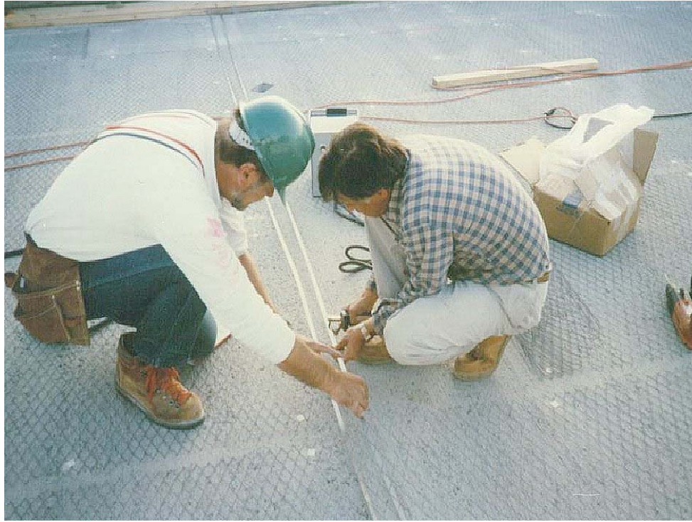
Figure 9.1 Titanium mesh anode system
