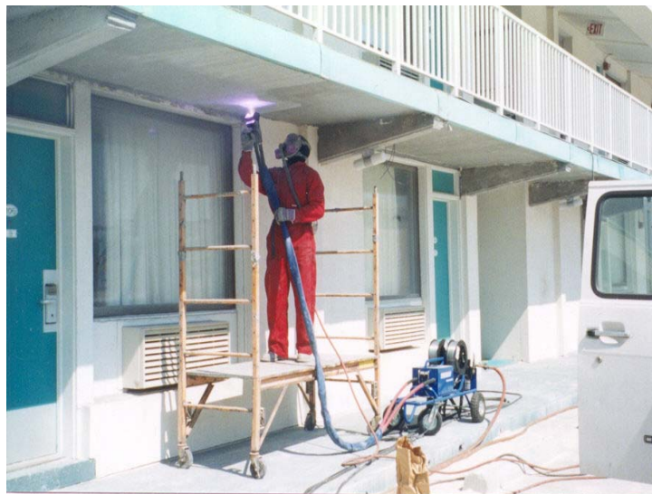
Figure 9.4 Arc spray application of galvanic anode
