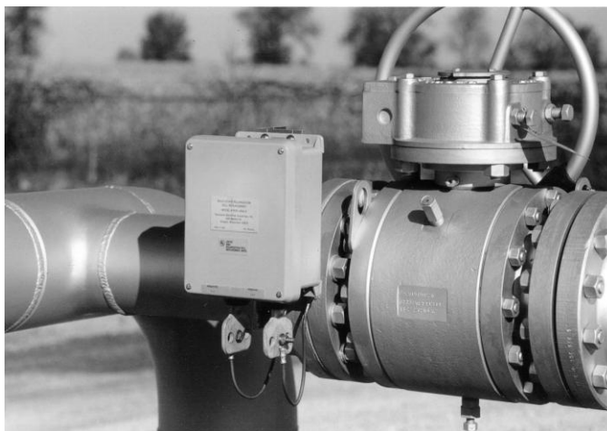
Figure 7.24 Semiconductor Device for AC and High-Voltage Fault Control (courtesy of Dairyland Electrical Industries)
