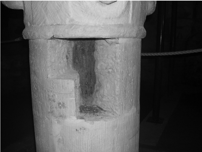
Figure 2.6 Damage to the eleventh-century Saxon stones in the vault at Gloucester Cathedral due to corrosion of the internal steel cores, which had been installed in the twentieth century.
