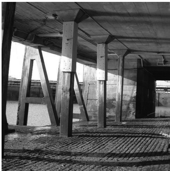
Figure 5.4 A jacketed zinc galvanic anode system applied to columns on a jetty in the Channel Islands, United Kingdom.
