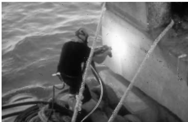
Figure 5.5 Thermal-sprayed zinc being applied to a bridge substructure in the Florida Keys in the 1990s.
