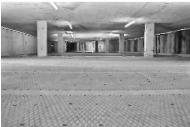
Figure 12.9 Anode installation on the first basement level.
