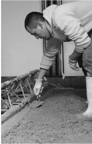
Figure 12.10 Casting of the PCC onto the floors to embed the anode mesh.
