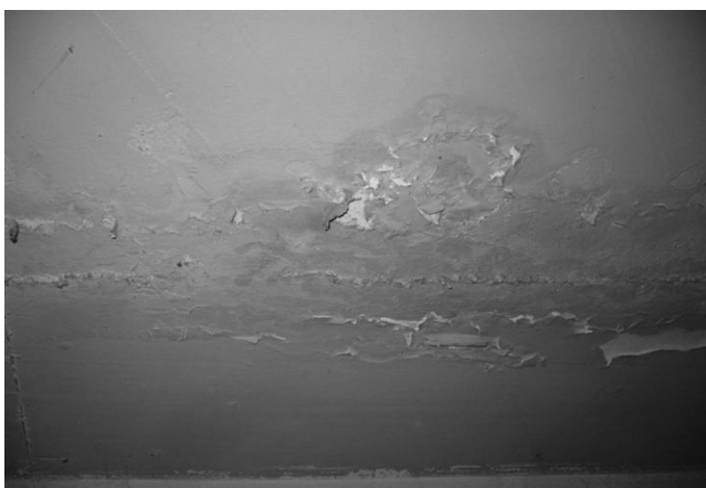
Figure 12.4 Damages and signs of moisture on the ceiling above first basement floor.
