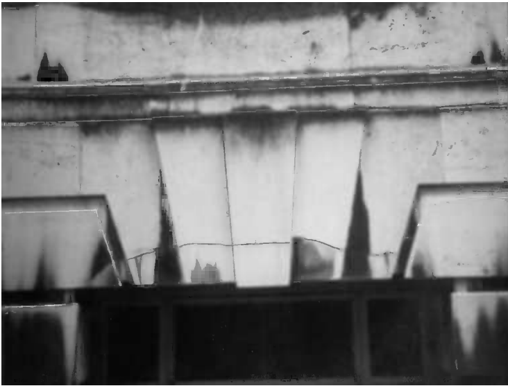
Figure 2.10 Practical example of the damage to steel framed construction as illustrated in Figure 2.9.
