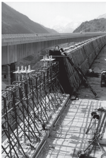
Figure 9.5 CP integration to new bridge safety barriers.
