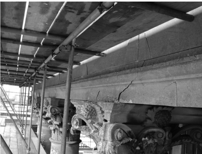
Figure 2.3 Typical damage to the original stonework of the architrave at Dodington House caused by water ingress and corrosion of embedded cramps.
