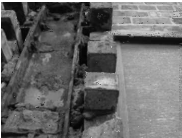
Figure 2.15 Damage to a vertical brick column due to corrosion and expansion of the steel frame.
