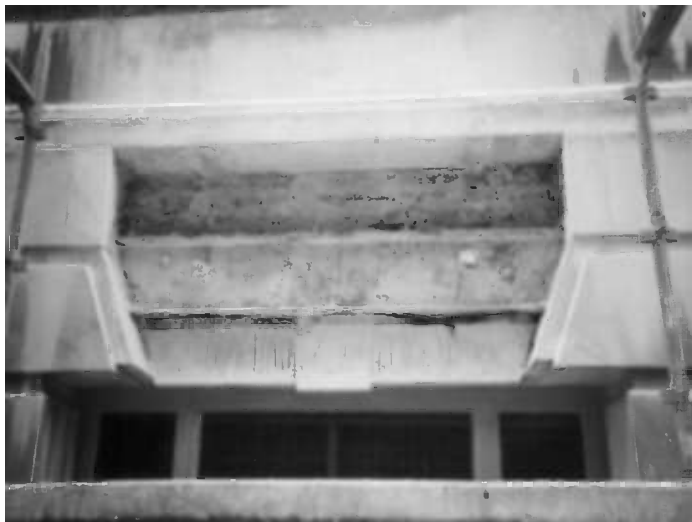
Figure 2.11 Opening up the steel framed construction to reveal the corroding steel beam.
