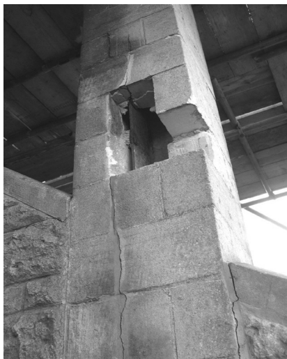
Figure 2.14 Cracking of the vertical pillars to a cricket pavilion at Downside Abbey and School, Somerset.
