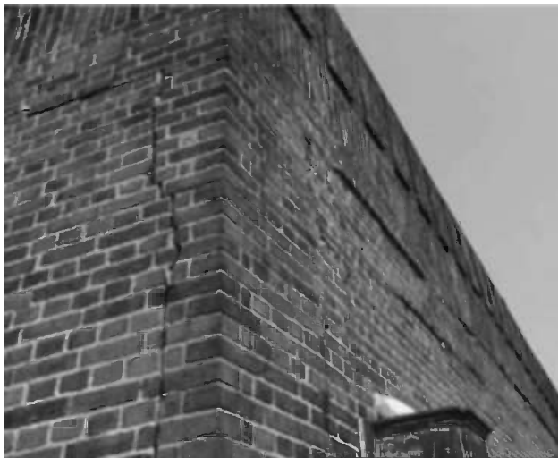
Figure 8.1 Vertical cracking caused by corrosion of the steel frame columns on a large, 1930s built brick building.
