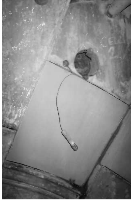
Figure 8.3 Damaged stones have been replaced before the cathodic protection contractor arriving on-site. A core hole is therefore required to make a connection to the steel and to install a reference electrode.
