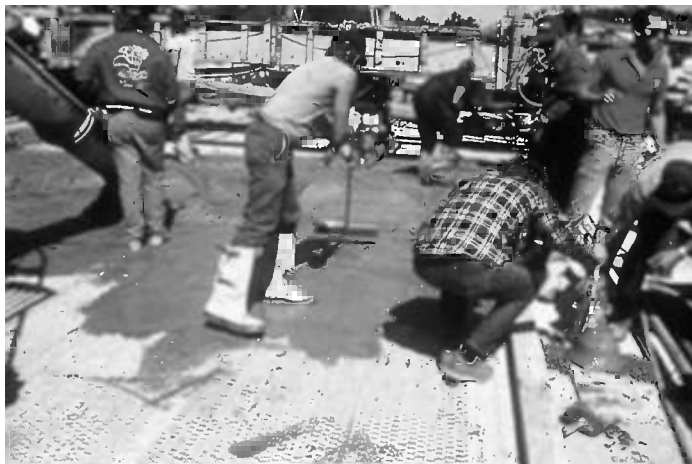
Figure 5.1 Early application of a mesh and overlay anode system on a U.S. bridge deck.
