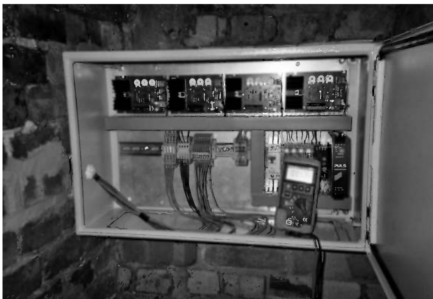
Figure 11.2 A simple manual impressed current cathodic protection power supply with four zones adjusted by the potentiostats at the top of the cabinet.
