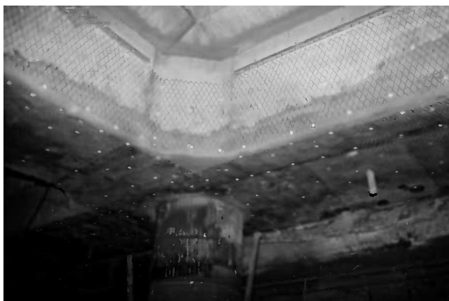
Figure 9.1 Kwai Chung jetty.
