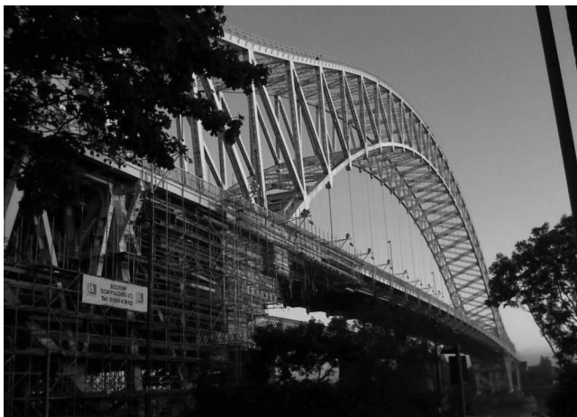
Figure 12.14 Silver Jubilee Bridge.
