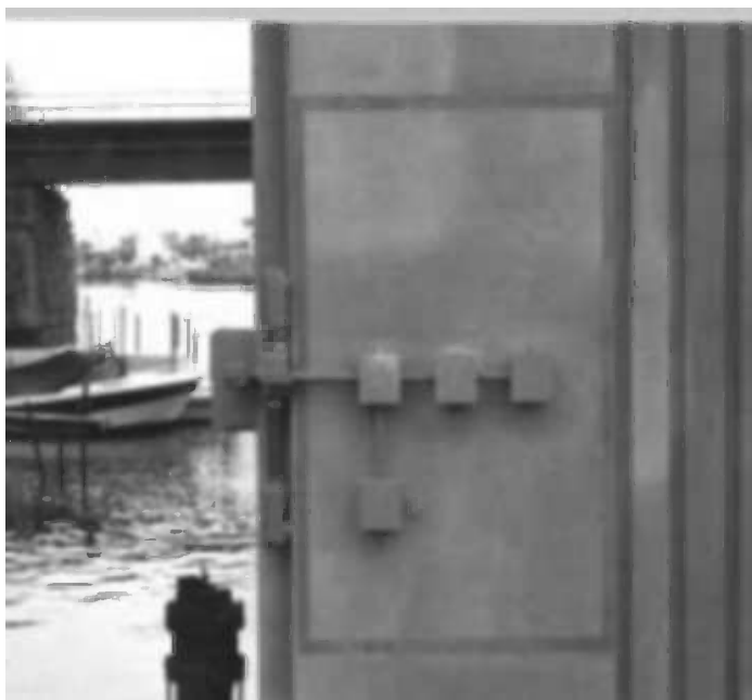
Figure 11.11 A window for current and reference electrode potential monitoring in a Corrospray™ Al-Zn-In thermal sprayed anode system on a marine bridge. (From Daily, S. F. and Green, W., Galvanic cathodic protection of reinforced and pre-stressed concrete using CORROSPRAY™ a thermally sprayed aluminium alloy, Corpro technical Library paper CP-51. 2007.)
