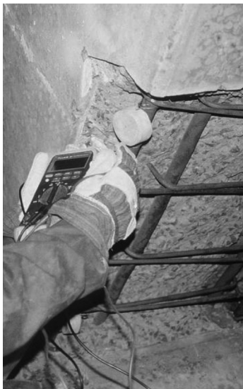
Figure 5.6 A galvanic anode in a patch repair to provide local protection around the repair and prevent the ‘incipient anode’ effect of corrosion around a repair.
