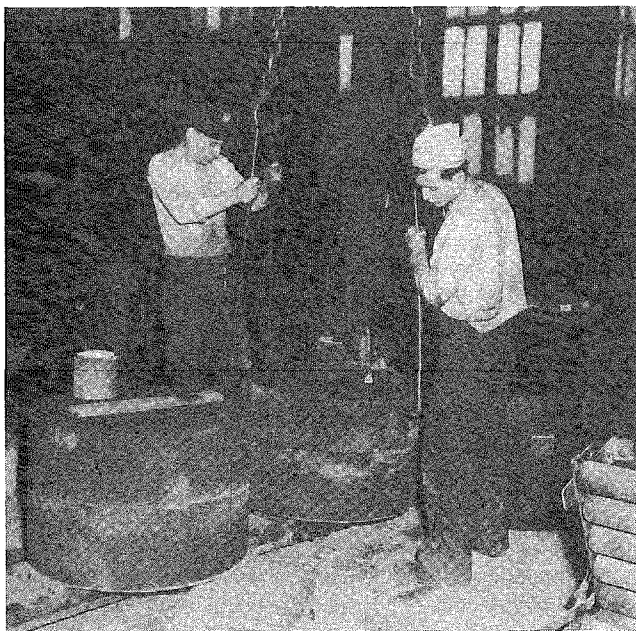
Fig. 4-3. Molds made of dry sand cores being inserted into a hinged door type of flask on a vertical machine in a steel foundry.
