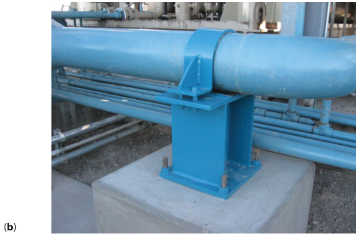
Figure 19.3 (a) Pipe clamp with liner material on the clamp ID and on pipe wedges. (b) Properly installed pipe clamp.
