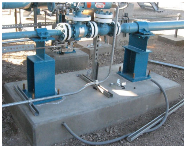
Figure 19.8 Correctly installed pipe clamps on concrete footing.
