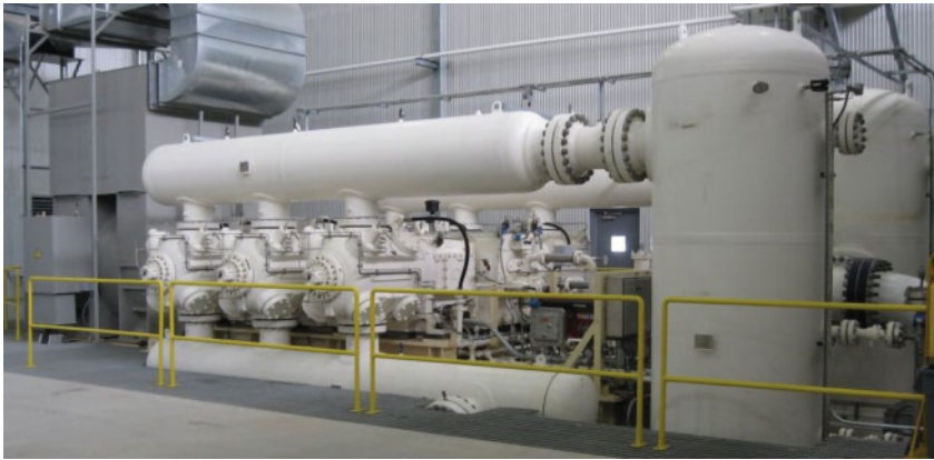
Figure A.6 Electric motor driven reciprocating compressor.
