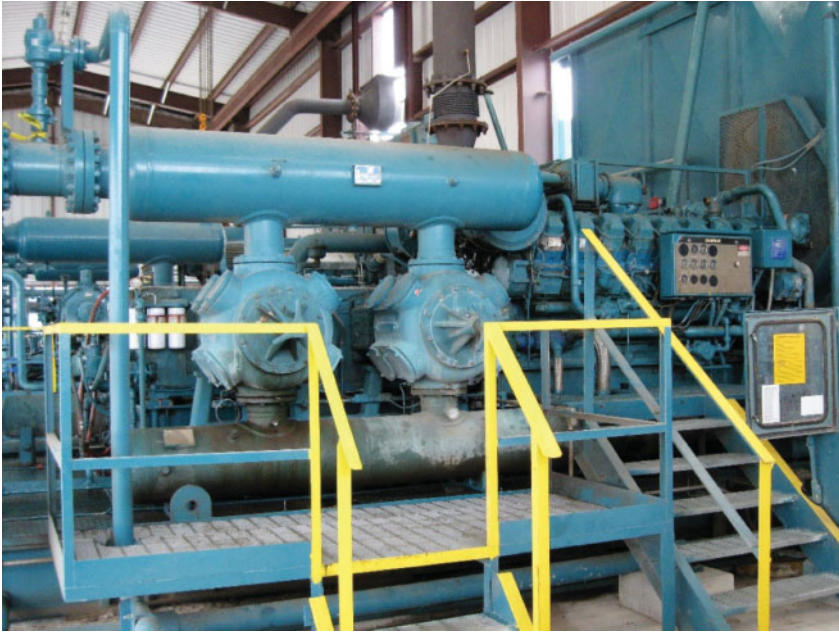
Figure 3.2 Reciprocating compressors' performance can be approximated using the adiabatic compression formula.
