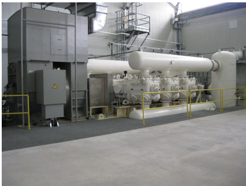
Figure 15.1 An electric motor directly coupled to a reciprocating compressor.
