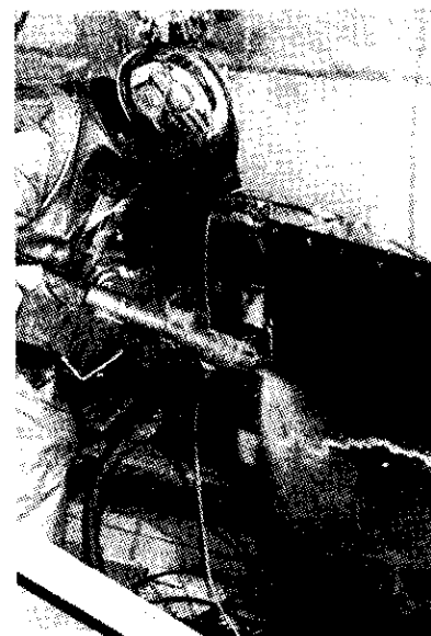
FIGURE 4-13. Ultra high pressure water cleaning of a 1/4 inch thick, 2-part fiberglass coating from a steel tank. Courtesy of Valley Systems Inc.
