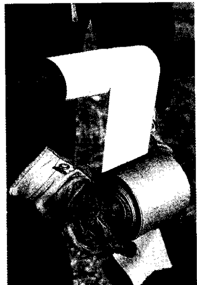
FIGURE 5-47. Proper overlap in tape application. Courtesy of the Trenton Corporation.
