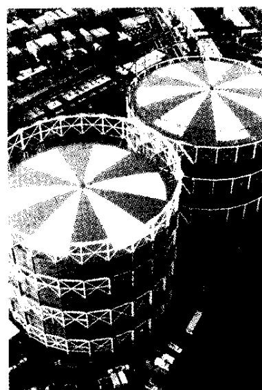
FIGURE 6-9. Special finish on tops of tanks to warn aircraft in the area. Courtesy of S.G. Pinney & Associates, Inc.
