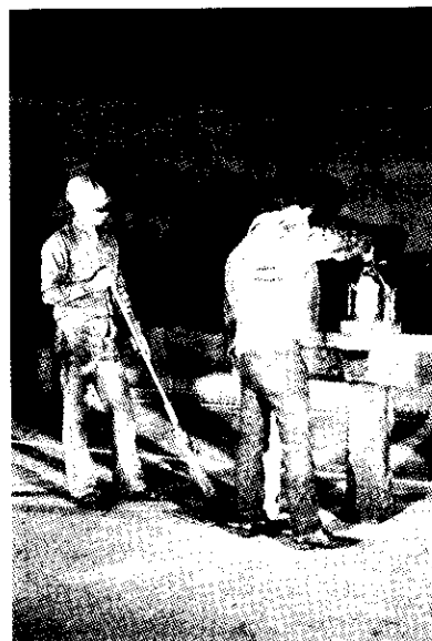
FIGURE 6-3. Unique structural features must be considered. Shown here is a floating roof with legs jacked up to apply FRP lining beneath. Courtesy of Amoco Chemicals.
