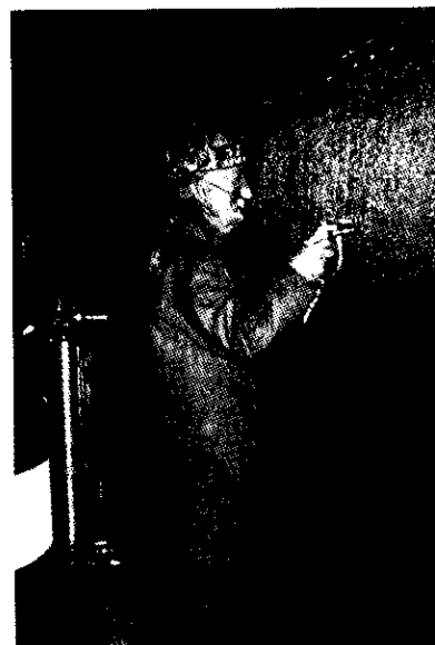
FIGURE 5-30. Spray application of a fluoroelastomeric coating. Courtesy of Colebrand, Ltd.
