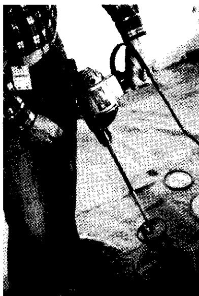
FIGURE 4-39. Mixing a one-component material. Courtesy of KTA-Tator Inc.
