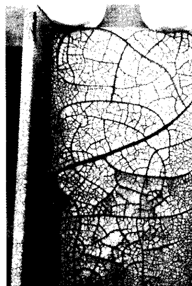
FIGURE 5-59. Mudcracking. SSPC file photo.
