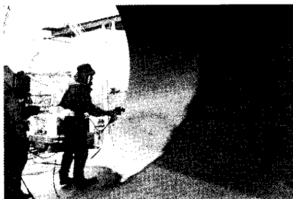
FIGURE 5-19. Applying a Class 6 epoxy modified coal tar pitch coating to the interior of a 20 foot diameter steel pipe. Courtesy of the author.
