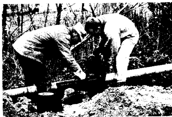
FIGURE 6-17. Manual application of a tape to a pipeline. SSPC file photo.
