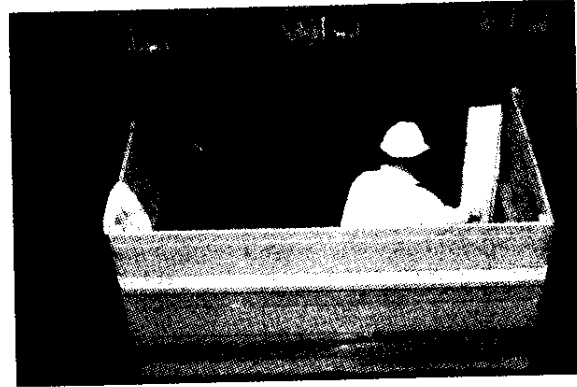
FIGURE 6-19. Use of a cofferdam to apply materials for immersion service. SSPC file photo.
