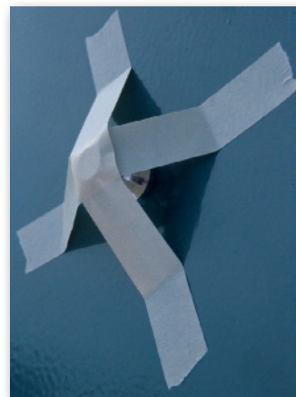
Use tape to hold pull stub in place
