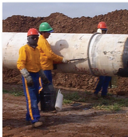
Holiday testing of pipeline using spring electrode
