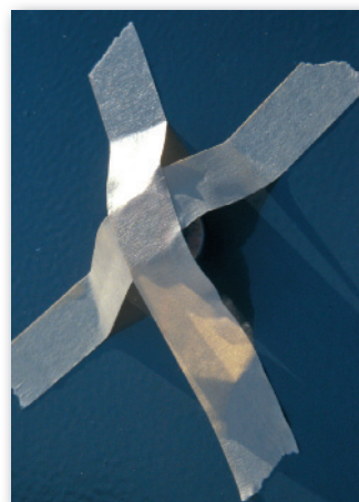
Use tape to hold the pull stub in place
