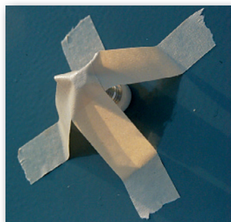
Use tape to hold pull stub in place
