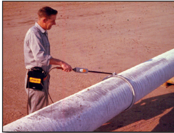
Holiday testing of pipeline using spring electrode
