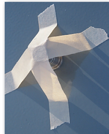
Use tape to hold pull stub in place
