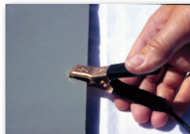
Attach ground wire clamp through coating to substrate
