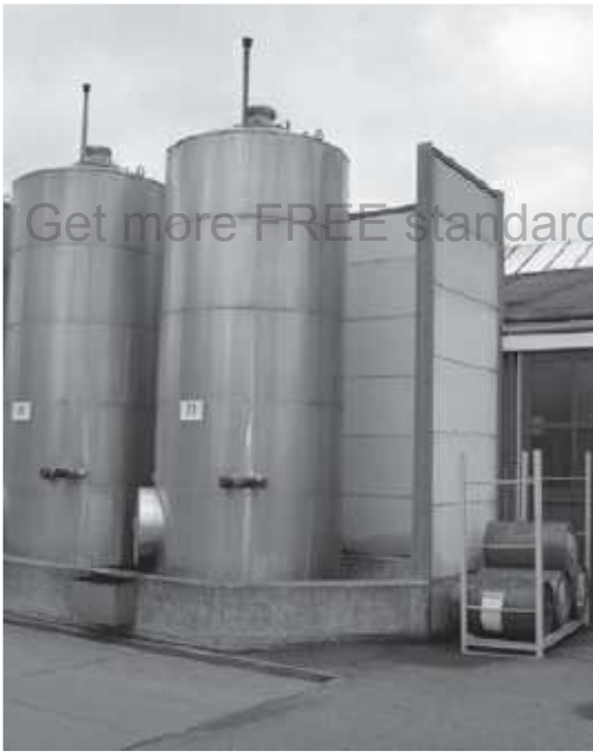
Figure 7.4: 20,000 litre tank storage for binders
