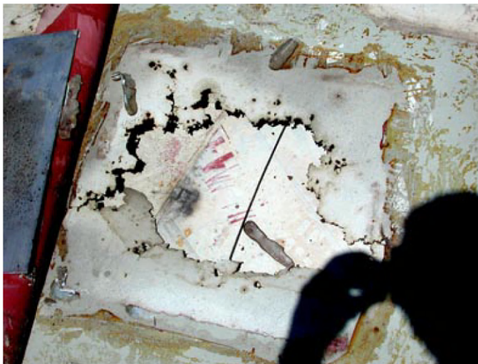
Fig. 3.15 Corroded roof of the gas oil AST after 5 years of service. (For a full color version of this figure, see the Color Section)
