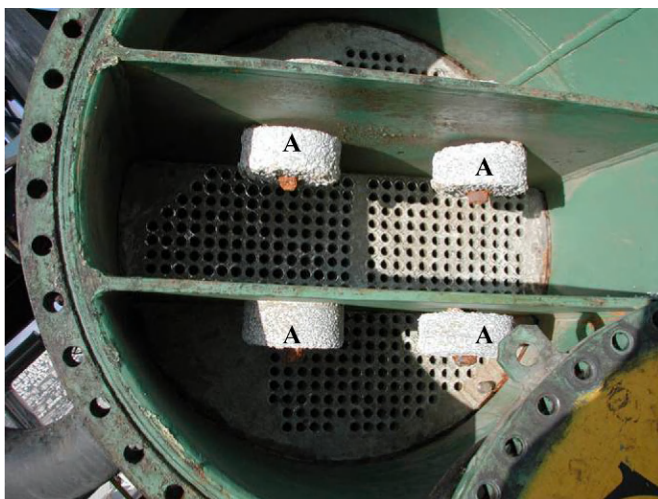
Fig. 4.8 Aluminum sacrificial anodes (A) installed on the inside of heat exchangers coated with epoxy paint (green). The cooling water flows inside the tubes. (For a full color version of this figure, see the Color Section)
