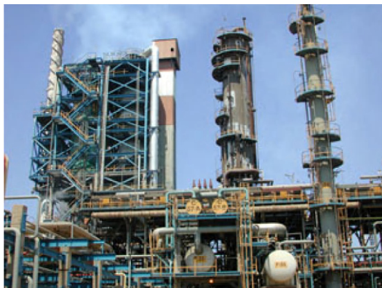
Fig. 3.3 Metallic structures and equipment in the atmosphere.
