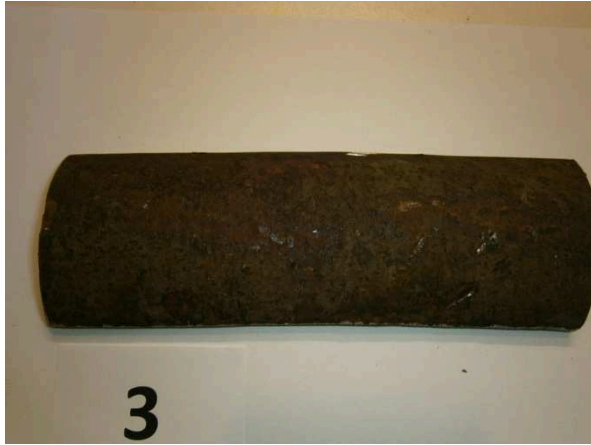
Fig. 6 Outer pipe surface (exposed to flue gases)
