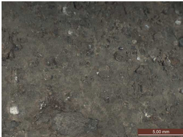
Fig. 8 Inner surface of pipe 3
