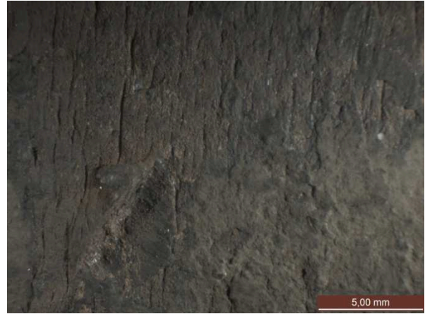
Fig. 7 Detail of corrosion layer (shown in Fig. 6) with minute cracks on pipe surface
