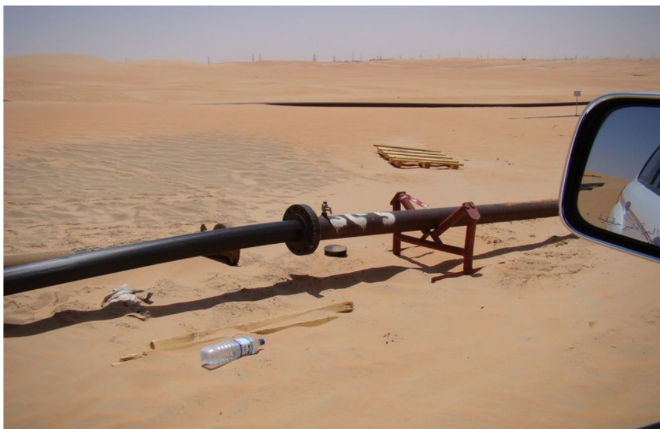
Figure 9.7 Field insertion of HDPE liner in a steel flowline. (see colour plate section).
