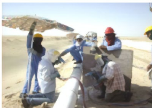
Figure 9.6 (a) Heat shrink sleeve coating on a weld joint in the desert; (b) application. (see colour plate section).
