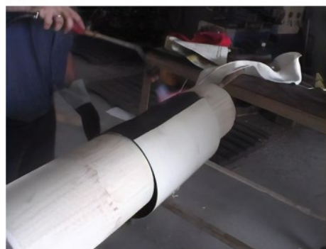
Figure 9.6 (a) Heat shrink sleeve coating on a weld joint in the desert; (b) application. (see colour plate section).
