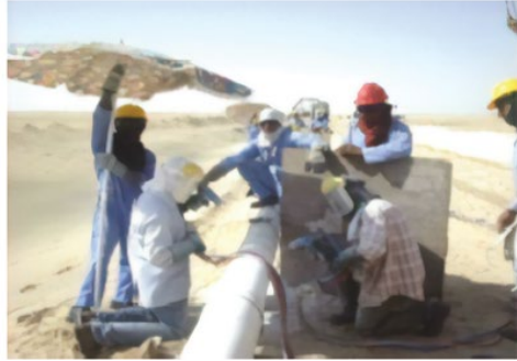
Figure 9.6 (a) Heat shrink sleeve coating on a weld joint in the desert; (b) application.
