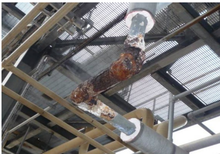
Figure 13.7 Isolated CUI of piping with expanded perlite insulation. (see colour plate section).
