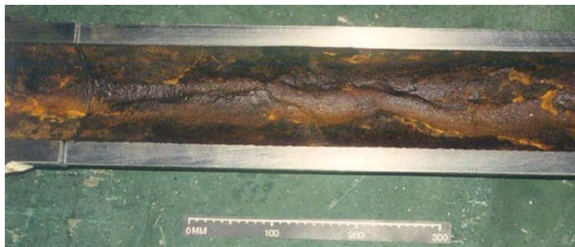
Figure 11.3 Groove corrosion promoted by microbial activity. Source: [2].
