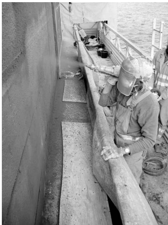
Figure 7.14 Conductive mortar anode applied to a marine bridge substructure.
