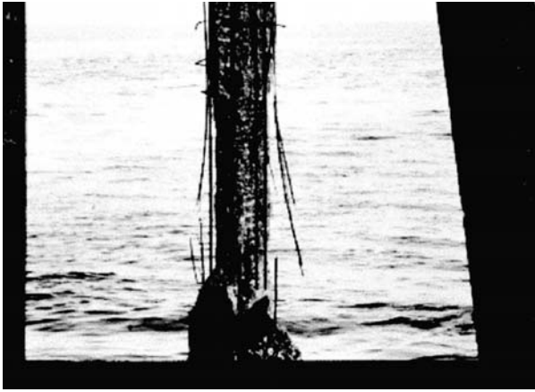
Figure 6.10 Pre-tensioned tendons corroded through three years after encasement from Rapa and Hartt (1999). Courtesy NACE International 1999.
