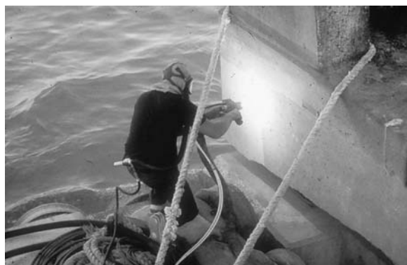
Figure 7.5 Thermal sprayed zinc being applied to a bridge substructure in the Florida Keys. Courtesy Florida DOT.
