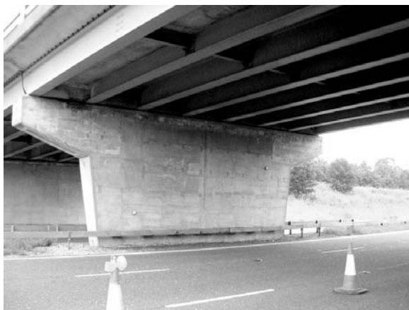
Figure 7.10 Thermal sprayed zinc applied to the leaf piers of Golden Fleece Interchange on the M6, UK. Probe anodes are applied to the cantilevered ends, the bearing shelf and the diaphragms between the longitudinal steel.
