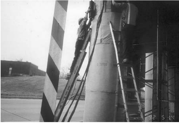
Figure 7.21 Geotextile blanket anode system being installed on a bridge column in the SHRP ECE trials (Bennett et al. , 1993a, Acknowledgement Transportation Research Board).
