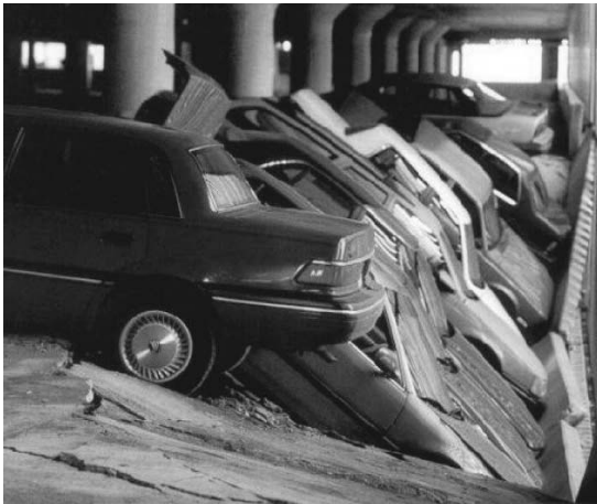
Figure 10.1 Collapse of the cantilevered section of a multi-storey car park in Syracuse, New York State due to deicing salt induced corrosion (Simon, 2004). Courtesy NACE International 2004.
