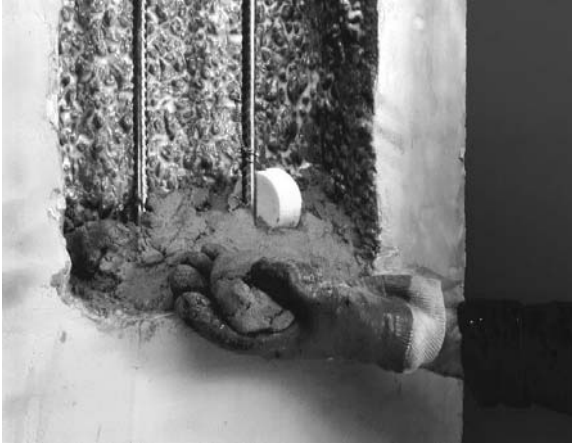
Figure 7.7 Installation of a galvanic anode in a patch repair to prevent incipient anode induced corrosion around the repair. Courtesy of Fosroc Ltd.
