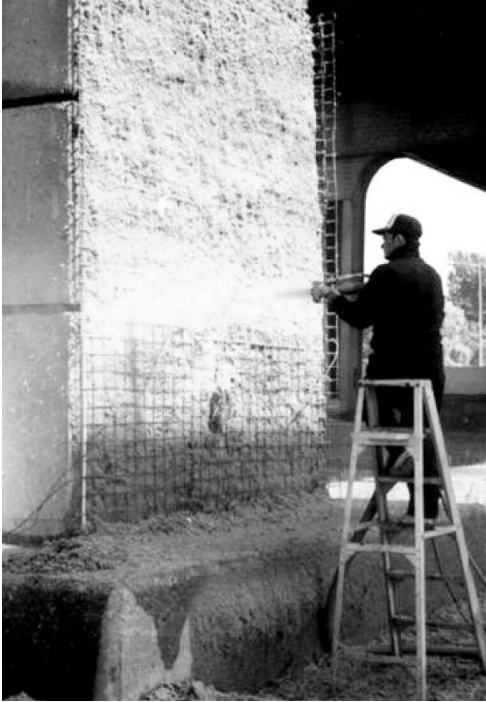
Figure 7.20 Electrochemical chloride extraction being applied to the Burlington Skyway Ontario, Canada 1989, using cellulose fibre over a mild steel mesh. Acknowledgements Jack Bennett.
