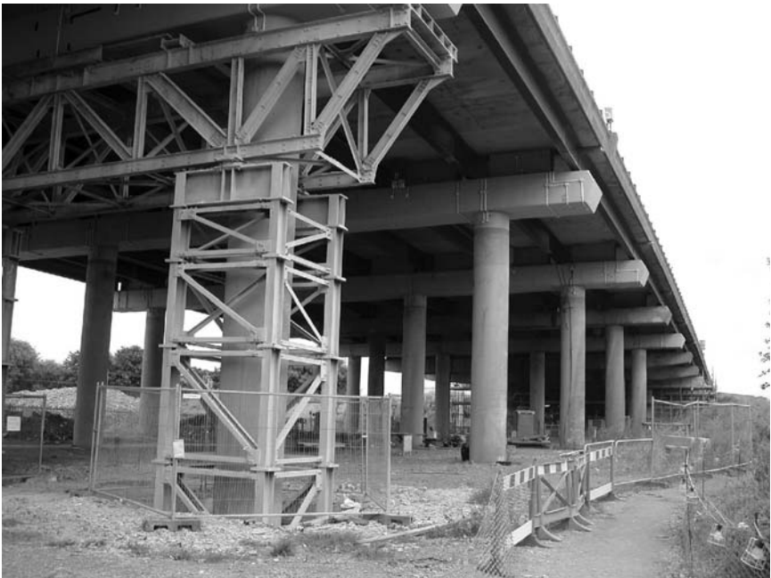
Figure 4.1 Structural support system on the Midland Links Motorway elevated section (Junction 9 M6) prior to repair. The support system is jacked up to take some of the load while concrete repair is undertaken. Conductive coating cathodic protection systems can be seen on subsequent cross heads. Courtesy of Kevin Davies, Corrosion Consultant, taken December 2005.
