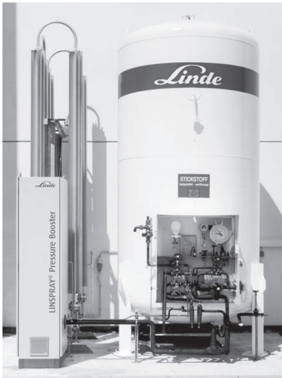
12.4 Liquid nitrogen supply by the Linde Gas Company.
