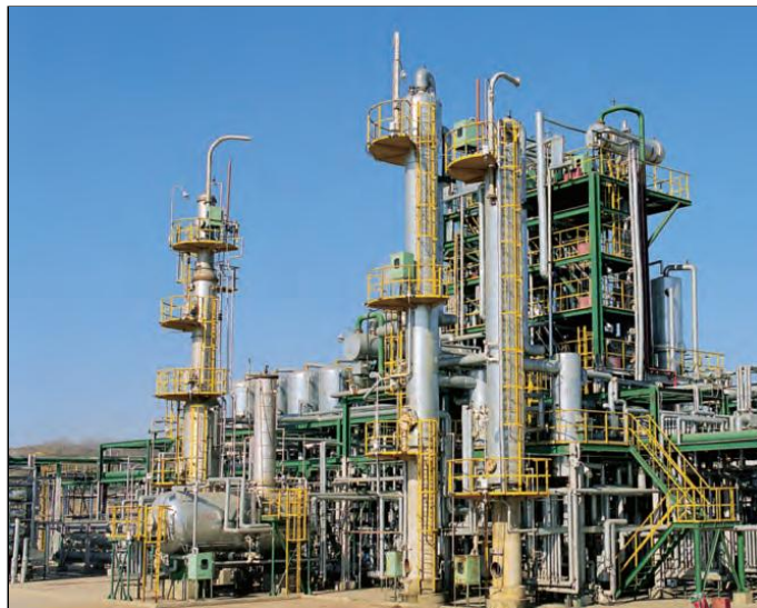
(Copyright Sulzer Chemtech Ltd., Switzerland)
