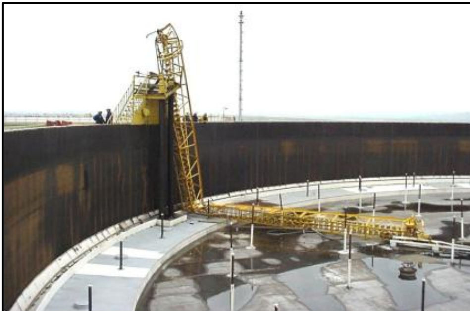
Figure 12 Effects of mal-operation, product change or severe weather on ladder stability
