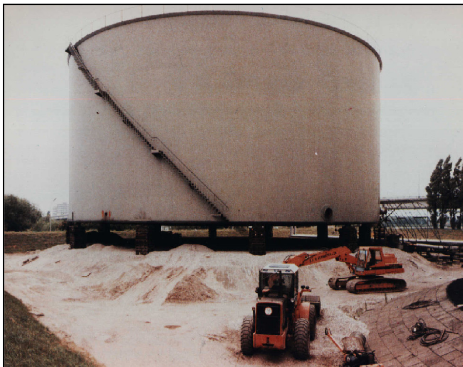
Figure 41 A 36 metre diameter tank jacked up 2.5 metres above the foundation
