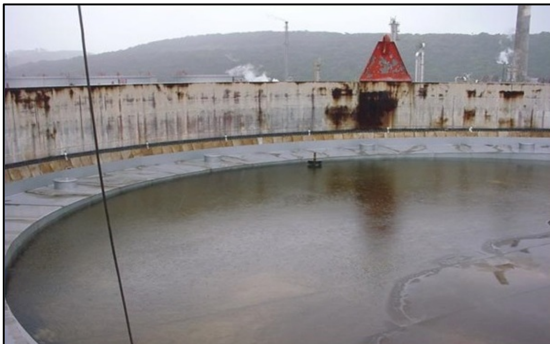
Figure 90 Example of effects of burping
