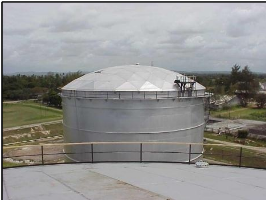
Figure 92 Typical geodesic aluminium dome on a fuel tank
