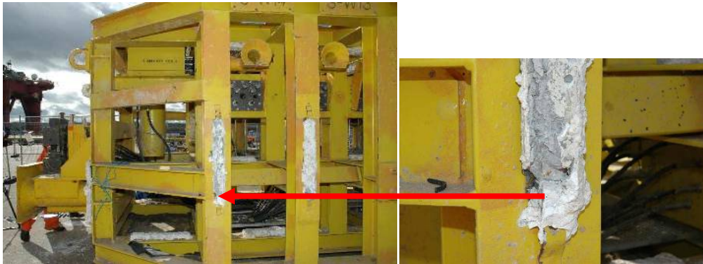
Figure 4 Subsea umbilical termination unit recovered after 10 years subsea, showing extensive wastage of the aluminium anodes but no corrosion of the steel structure
