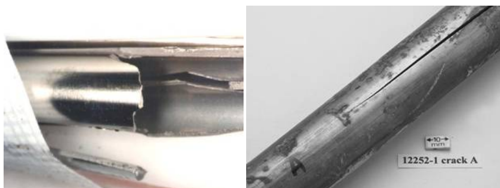
Figure 23 Brittle failures of superduplex stainless steel umbilical tubing
