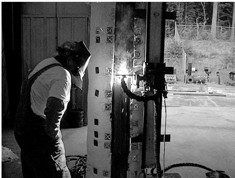
Figure 2-9 Seam Weld Pipe Overlay Demonstration Mockup #2
