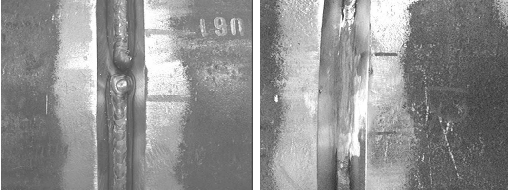
Figure L3-3. Start and stop location at tack weld before and after preparation for hot pass.
