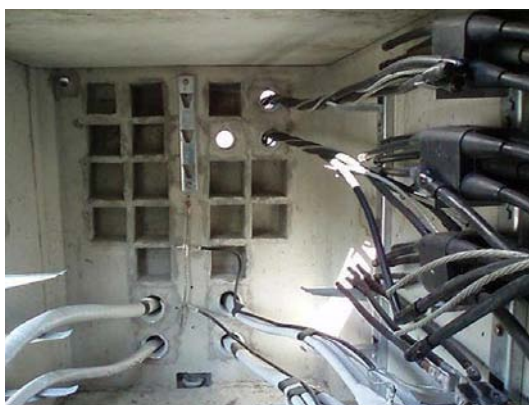
Figure 10.8 Manholes are an example of confined spaces.
