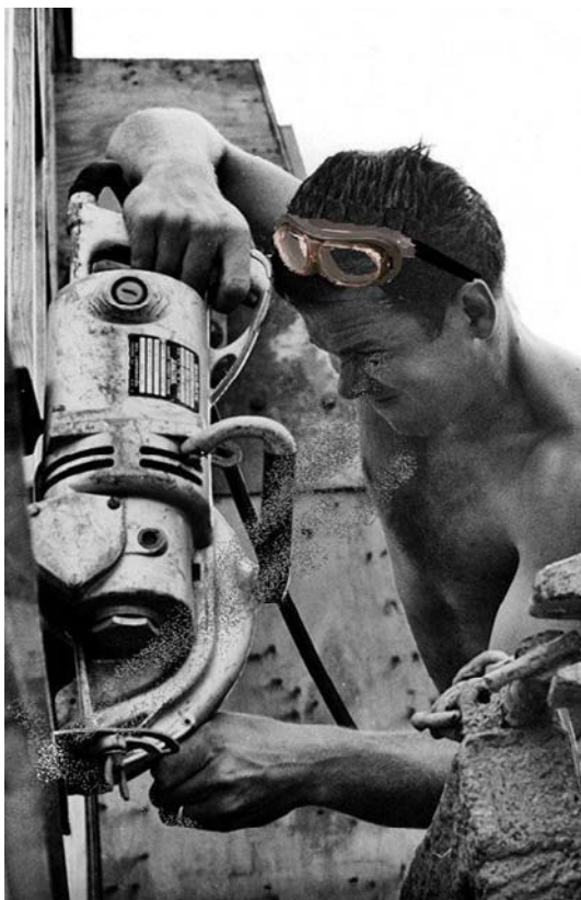
Figure 10.3 If eye protection does not fit properly, workers are not likely to wear it as they should to comply with OSHA requirements.
