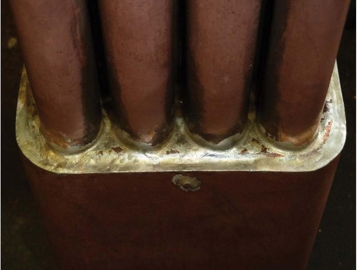
Photo 21 Detail of tube to tubesheet joints, silver soldering complete, boiler side.
